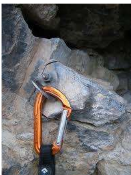
Example of a Sub-Standard Anchor. While the anchor assembly complies to EN 959, the fractured rock becomes the weak point.
