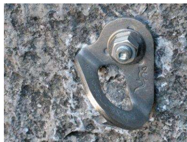
Example of a solid Fixed Anchor safe for use. Rock is solid with no fractures; hanger sits flush with the rock and cannot spin.
