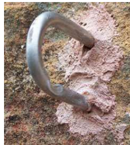
Worn and poorly placed U-bolt. Anchors with any visible signs of wear should be immediately replaced.
