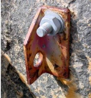
Homemade hanger on mild steel bolt. All bolts and hangers should be stainless steel and hangers should conform with EN-959.
