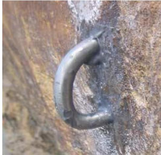
Note that there is at least 16mm clearance to allow carabiners to rotate freely and load correctly
